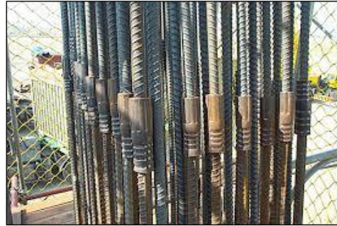
Couplers connecting column bars
