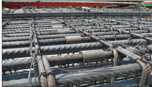
Threaded couplers joining bars of a RC slab
